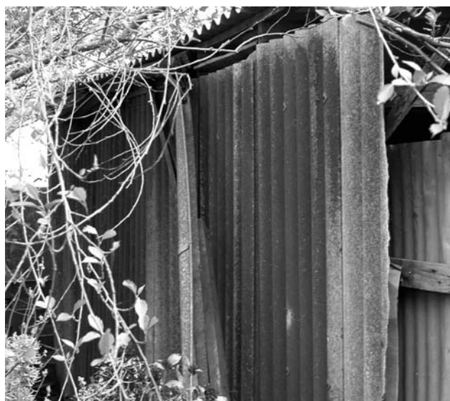
Asbestos cement sheeting on the wall and roof of a shed.
