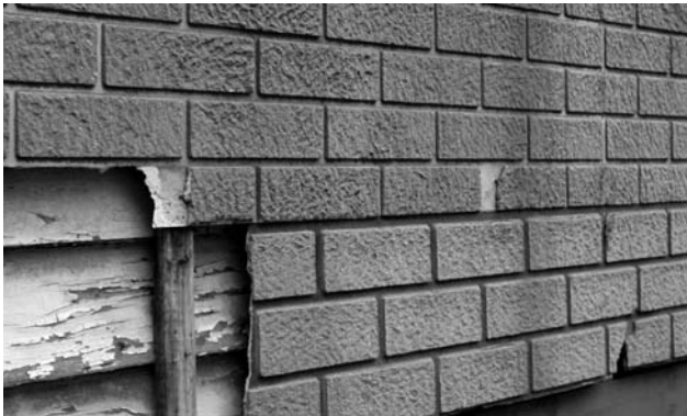
External cladding containing asbestos.
