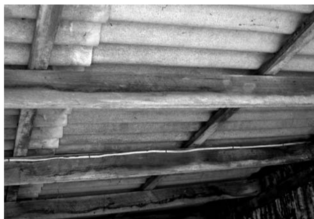
Underside of asbestos cement roof sheeting.
