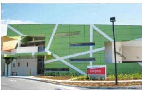
Robina Hospital Emergency Department
