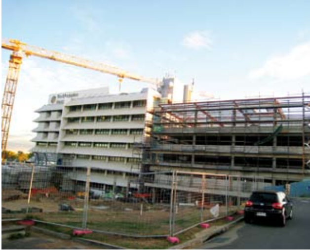
Redevelopment at Rockhampton Hospital.
