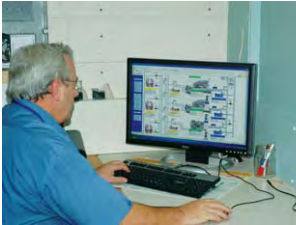
An engineering-maintenance manager using the building maintenance system installed at Hervey Bay Hospital.
