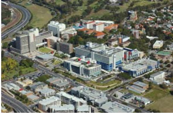
A recent aerial view of the hospital redevelopment.
