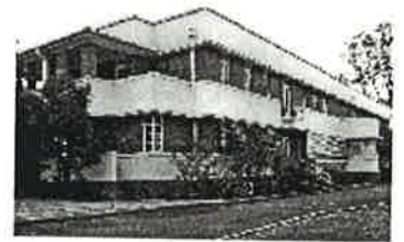
Staff quarters & administration block, Kingaroy Hospital
