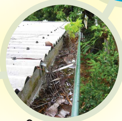
Gutters Clean regularly
