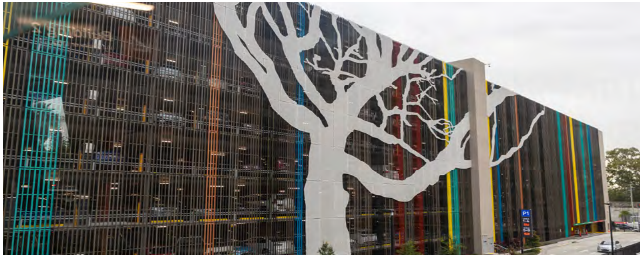
Louvreclad and MODE Design Corp, Logan Hospital car park facade, Our journey as one big family tree , 2021. Photograph: Queensland Health.
