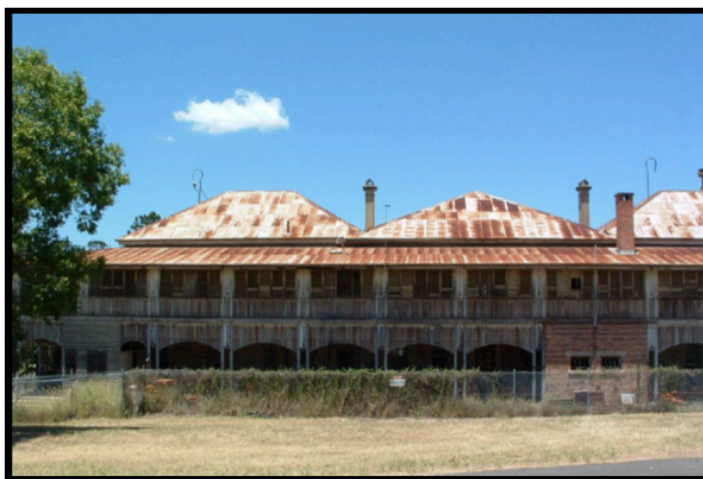
Wolston Park: Source Queensland Heritage Register
