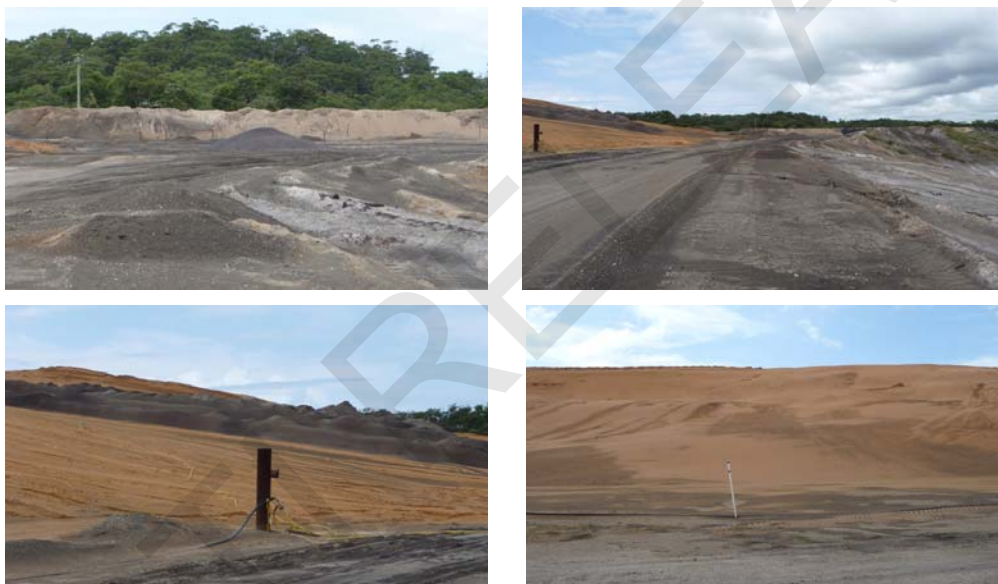
Figure A5 Tailings returned to North Stradbroke and covered with 10m of clean sand
